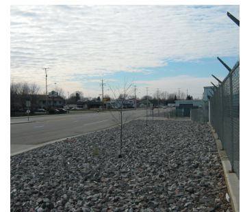
Looking West along Property line on Hwy. 23
